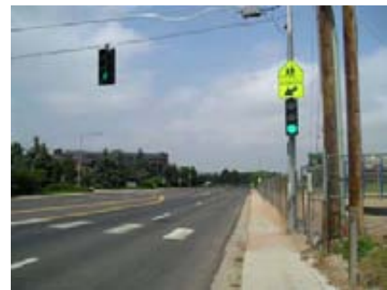
W. 88 th Ave Looking West Toward Yates
