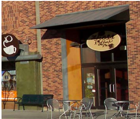
Bradburn Building Elements/Awnings
