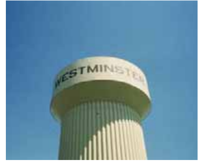
Above, the Hyrdopillar provides additional water storage for the city.
