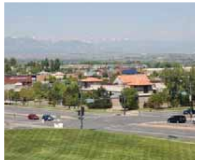
Future improvements to the roadway network will include a new Sheridan Boulevard bridge over US 36, new bike lanes and intersection improvements at various locations.
