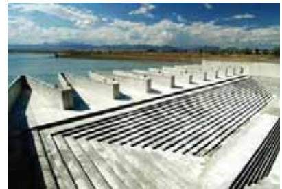
Standley Lake is the primary storage facility for the city's water supply, top. Bottom, the Labrynth Spillway, which is part of Standley Lake Dam.
