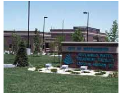
Big Dry Creek Reclaimed Plant.
