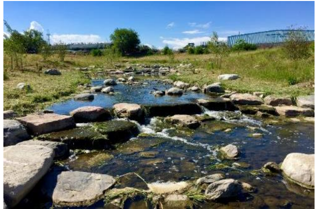
Boulder Drop Structures at Lowell Blvd.
