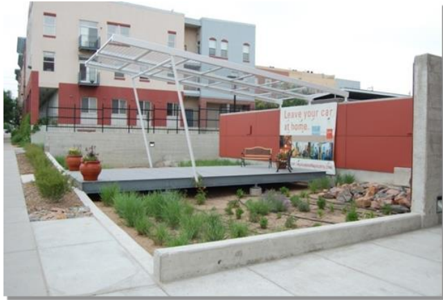
Photograph 3-A. This rain garden provides bioretention of pollutants, as well as an attractive amenity. Treatment should improve as vegetation matures.
