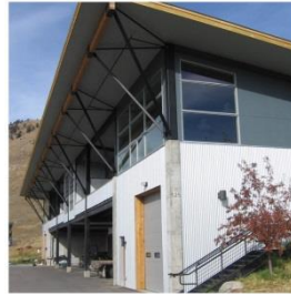
Small-Scale Industrial Warehouse
