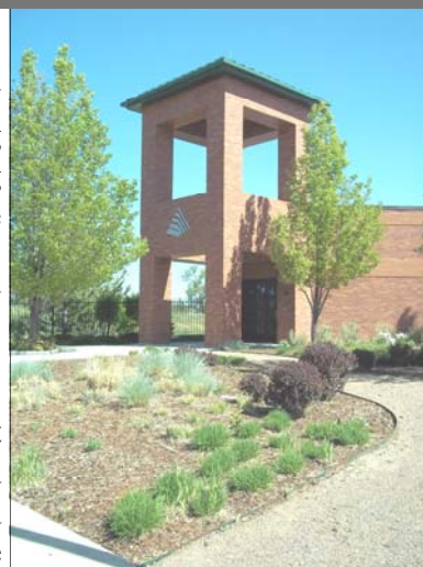
Northwest Water Treatment Facility
