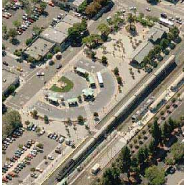
Multi-modal transit Station, Mountain View, CA
