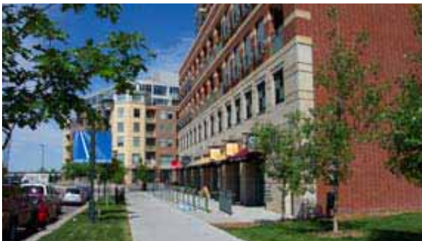
Treelawn and sidewalk treatment at mixed-use building
