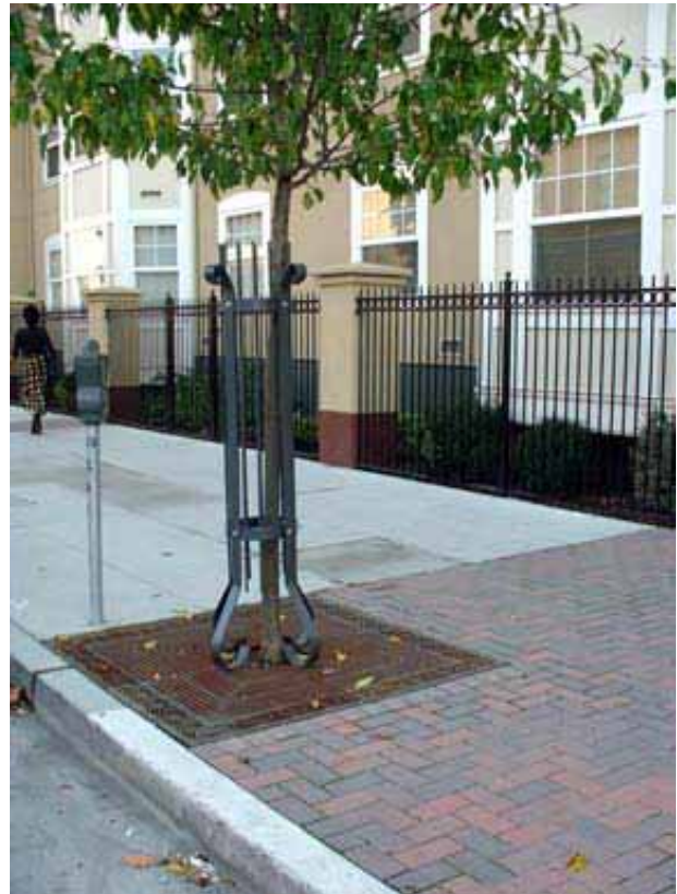
Tree grate, guard, and sidewalk paving
