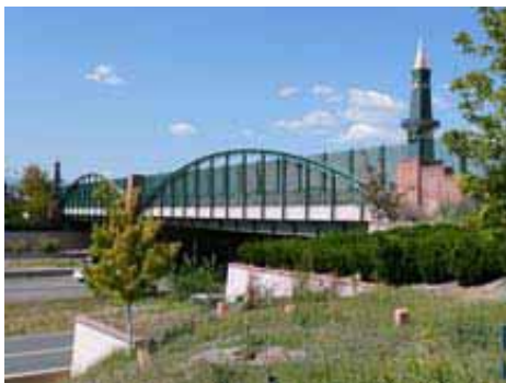
92nd Street Bridge at US 36 Westminster, CO
