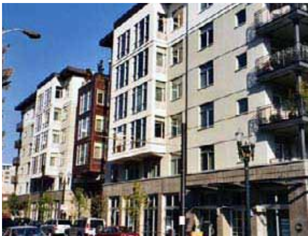
Mixed-use residential building
