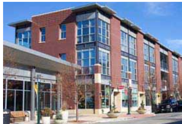
Mixed-use residential building
