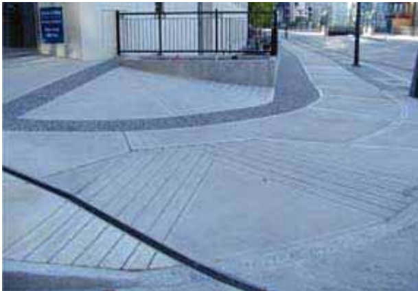
Special corner paving
