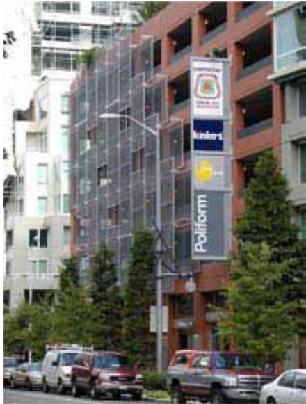
Parking structure, Seattle, WA
