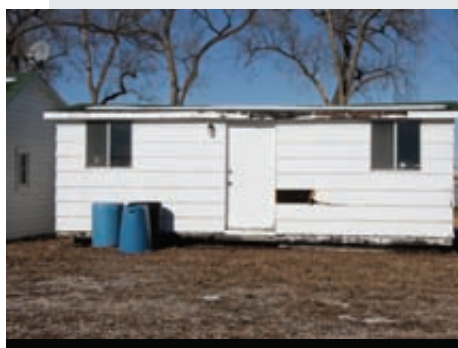
Images top to bottom: the caretaker's house, shop and garage, pump house, granary, and storage shed
