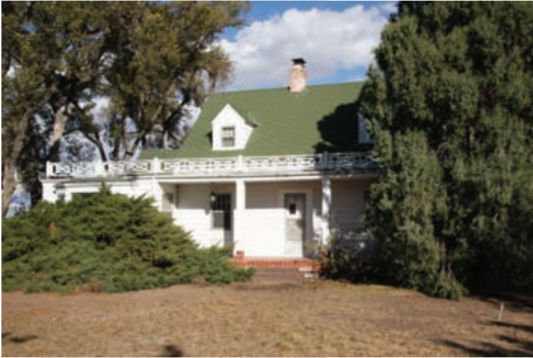
The main entry of Metzger farmhouse, where a circular drive was once located
