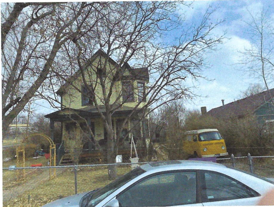
Front of house from the west side (Irving St)
