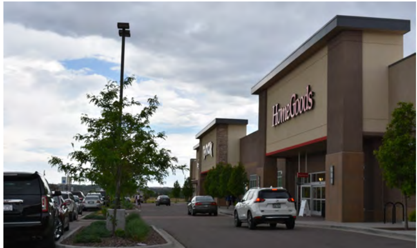
New development at Orchard Parkway and 144th Avenue
